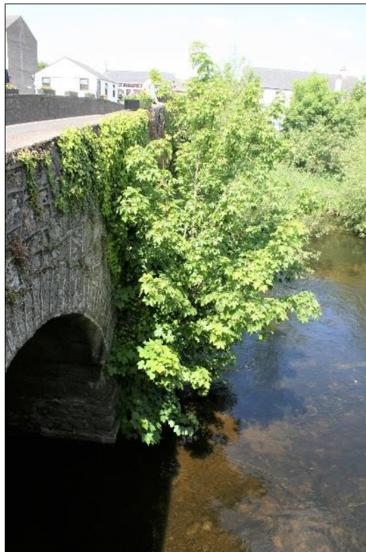
Plate 8: Sycamore tree rooted into pier on north-east elevation looking north-west
