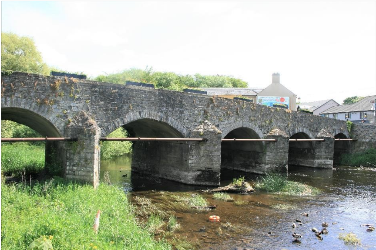
Plate 1: South-west elevation from west. Cement strap pointing and steel ducts interfere with visual integrity and pointing is likely to accelerate deterioration of masonry structure.
