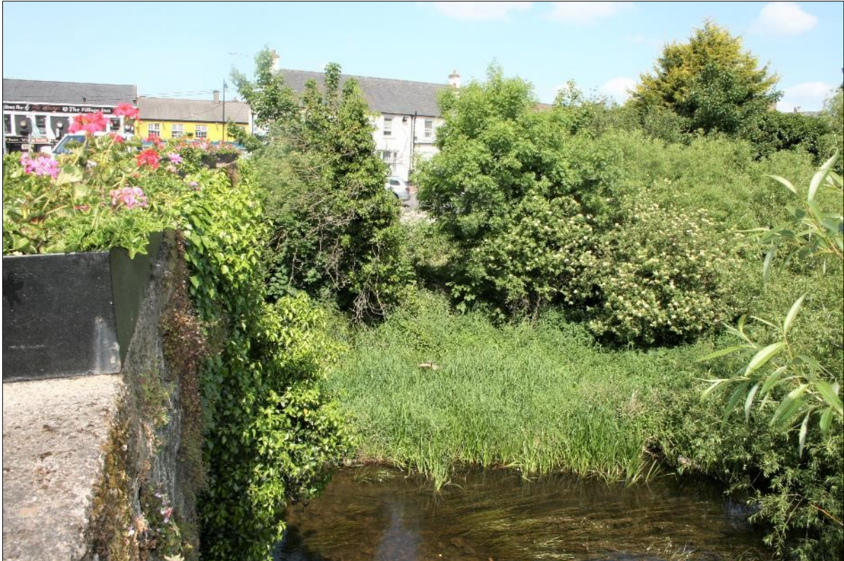
Plate 7: North-west side of north-east elevation showing extensive ivy and tree growth on structure and possible restriction of water floor through archway to north-west side.
