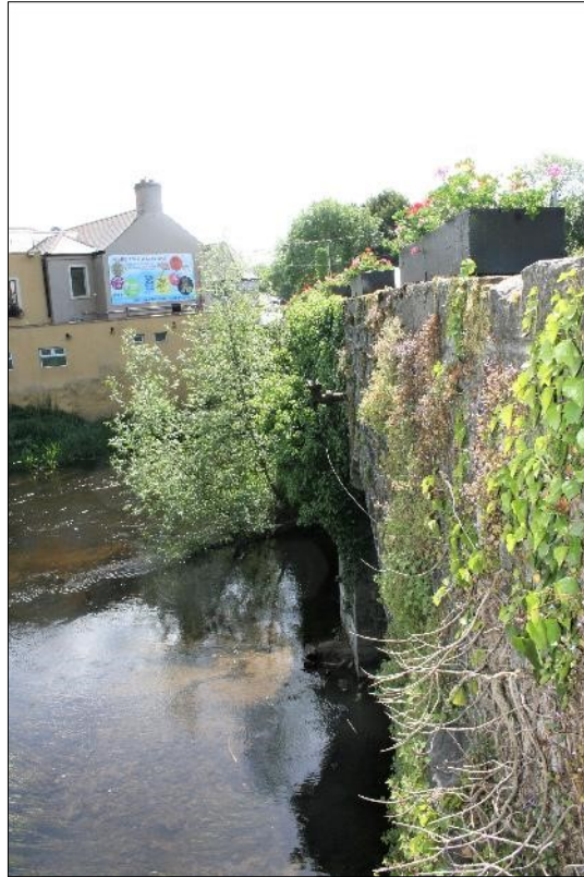
Plate 9: Tree rooted into pier and extensive heavy ivy growth on north-east elevation looking south-east
