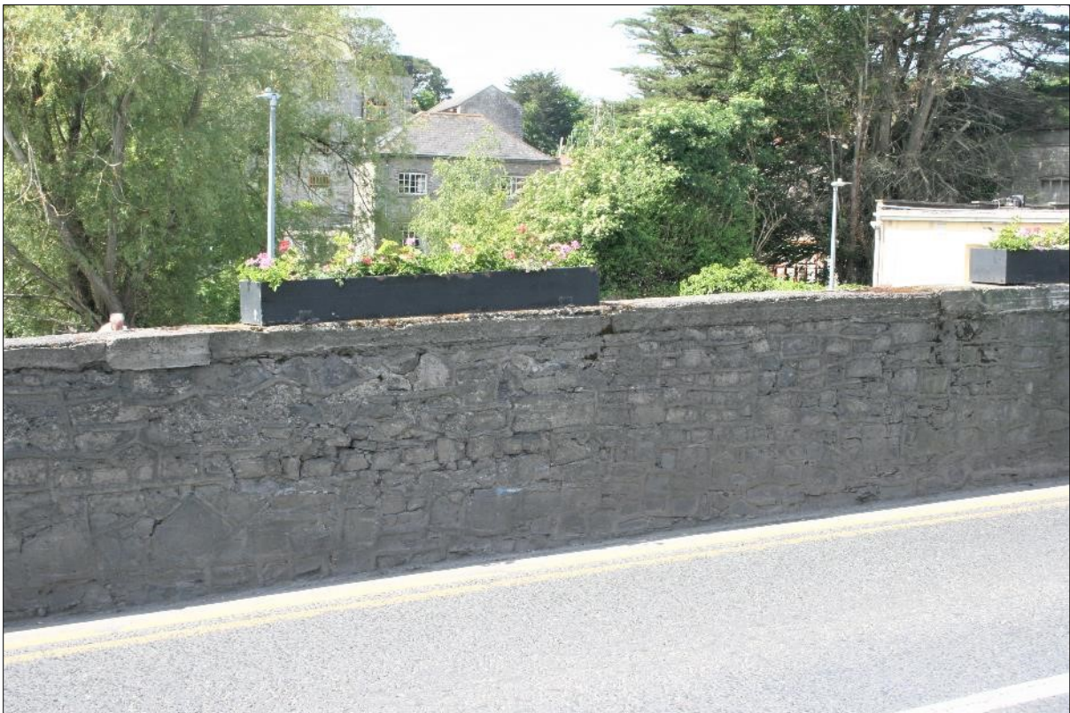
Plate 12: Loss of bedding mortar and later cement-rich pointing on interior of south-west parapet
