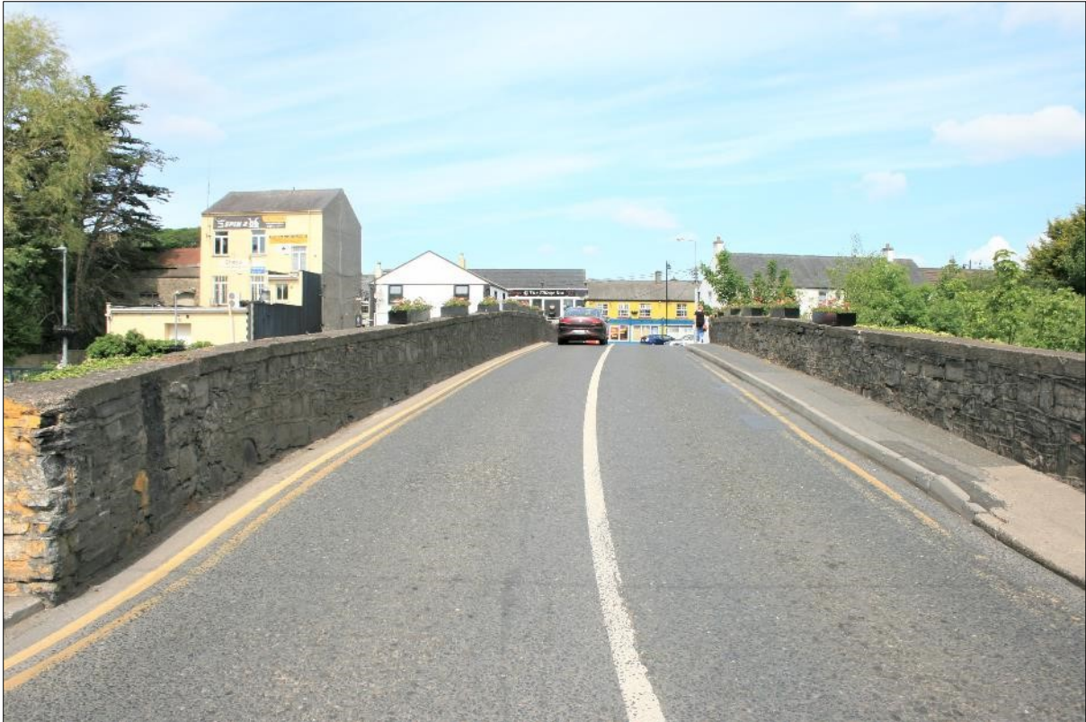
Plate 11: Roadway from south-east
