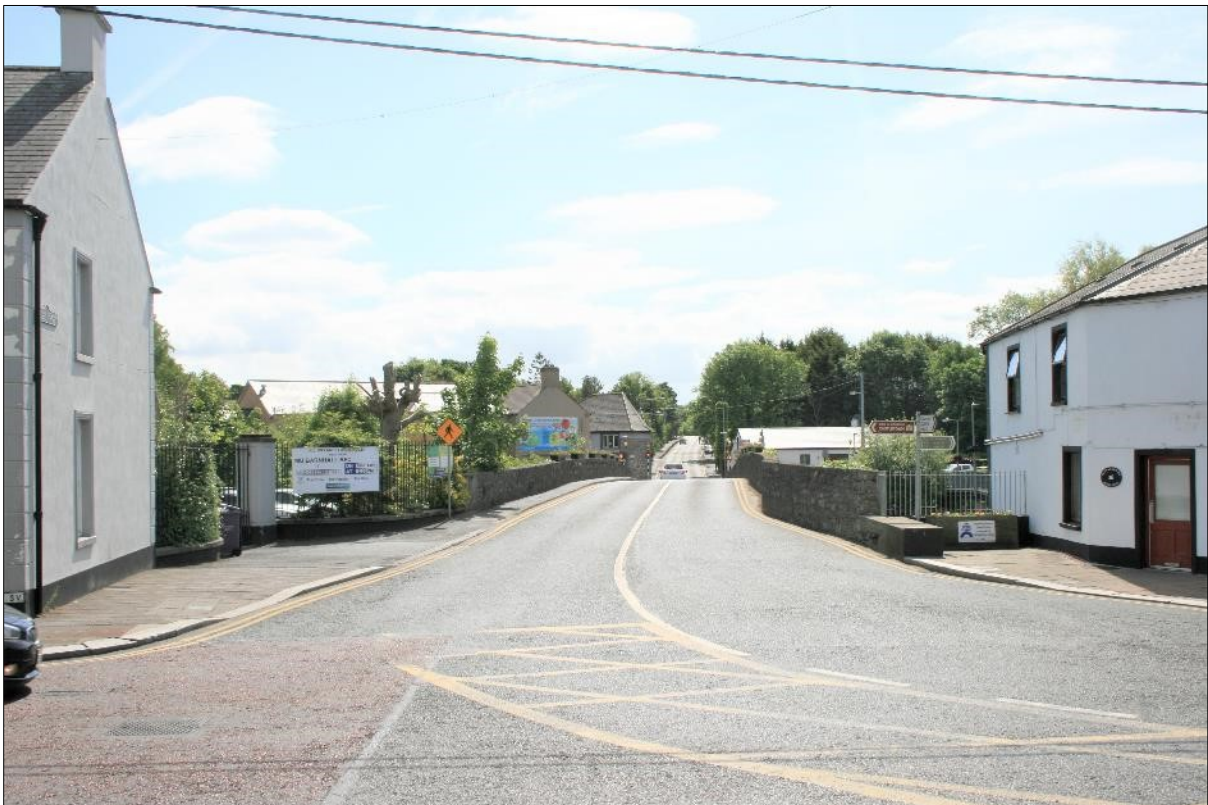
Plate 14: Roadway approaching bridge from north-west
