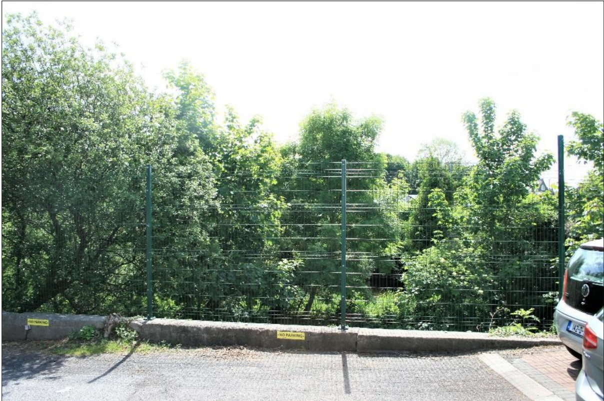
Plate 21: View to south-east across north-east elevation of bridge from car park of the former Bank of Ireland on Main Street.
