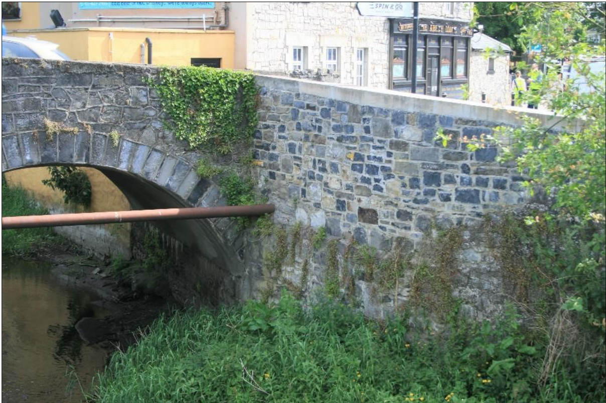
Plate 3: Re-built section to south-east wing wall adjoining bridge with poor bonding of stone, ie. long unbroken vertical joints extending over more than two stones. Localised ivy growth should be maintained to prevent deeper penetration by roots.
