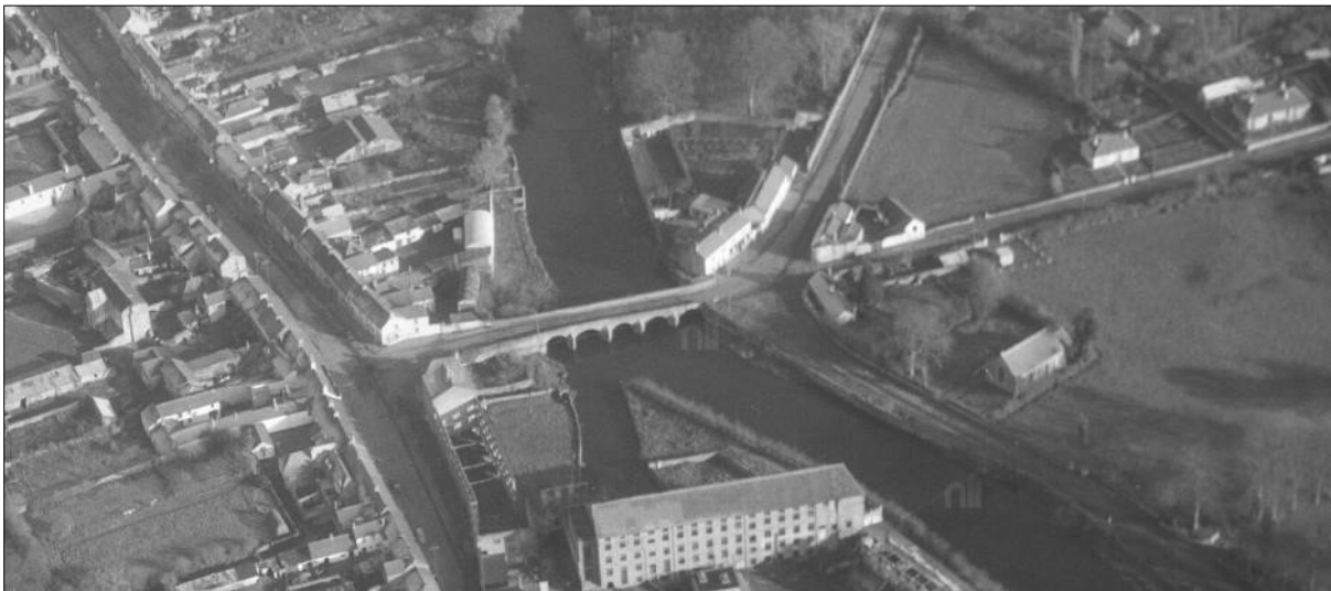
Figure 3: South-west elevation of the bridge, November 1956 http://catalogue.nli.ie/Record/vtls000737703
