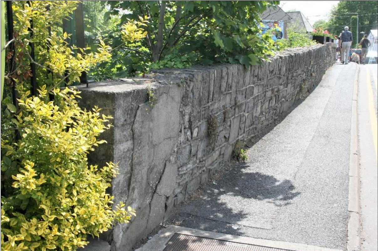
Plate 15: c.13m section of north-east parapet wall with vertically-bedded coping stones which is leaning inward towards road.
