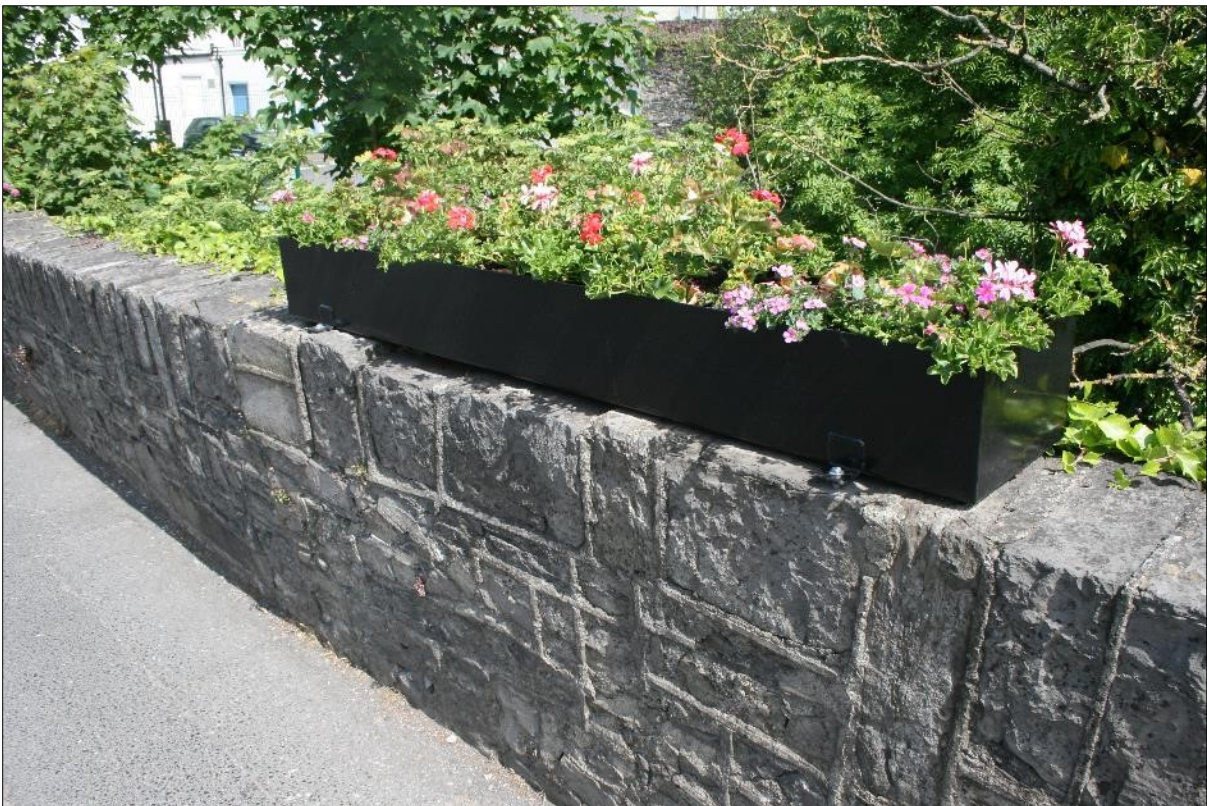
Plate 16: Fixings drilled into limestone capping close to edge of stones
