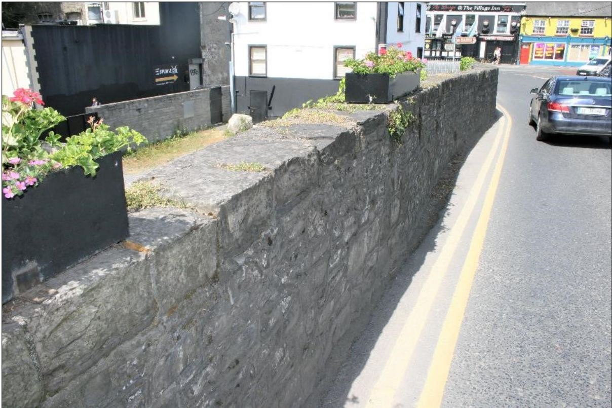
Plate 13: Detail of horizontal-bedded heavy limestone capping to south-west parapet
