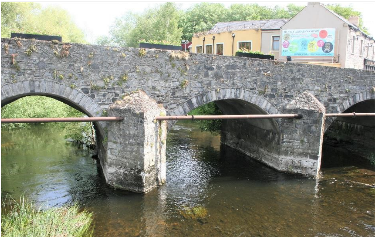
Plate 2: South-west elevation of south-easternmost pier (right) showing loss of pointing mortar from lower courses of masonry above water-line and wide open joints just visible to downstream side indicating scour erosion and loss of core material from pier.
